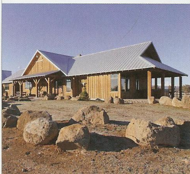
The house borrows from traditional Western ranch forms to respond to the regional climate.
